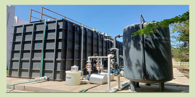
Water Treatment Plant (WRP) at TEN Coaching Depot aims at treating and reuse of waste water generated in the pit subjecting it to Physico-Chemical treatment by adding suitable Effluent treatment chemicals and to achieve treated effluent quality as prescribed by the TNPCB.
